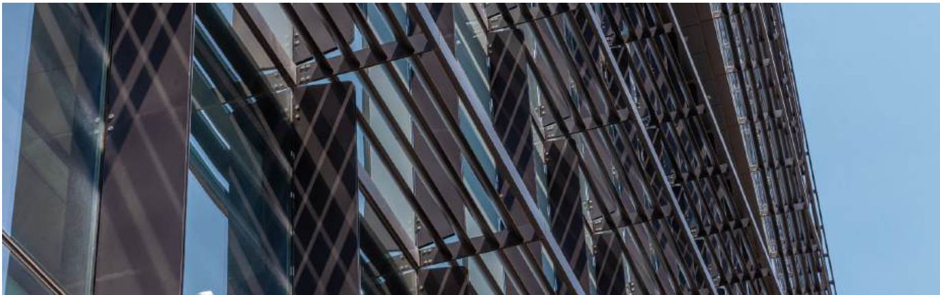
Cummins Indy Distribution Headquarters building in Indianapolis using AMPG's low profile sex bolts in its architecture.
